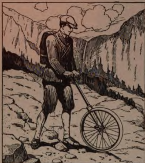
By Pushing a Bicycle Wheel with a Cyclometer before Him, a Pedestrian Measures the Exact Length of a Mountain Trail
